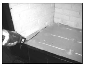
Figure 11.2. Using a saws-all, cut out the floor.
